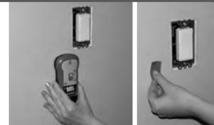
3. Place the flat side of mounting bracket (included) against the wall and align the thin side over the outside edge of the existing electrical box (opposite the stud side). Center the bracket to align the mounting screw height with existing switch, then trace the inside shape of the bracket on wall using a pencil or thin marker.
