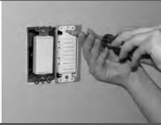
8. Attach a new (2 gang) or double gang Decora style wall plate over both switches to complete installation.
