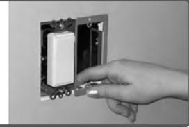
7. Position the DecoFlex RTS switch into mounting bracket aligning the screw holes. Ensure that the wire antenna remains as straight as possible behind the wall. Secure switch to mounting bracket with screws (provided).
