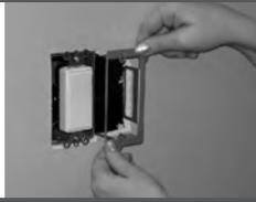
6. Carefully bend bracket tabs 90 degrees behind the dry-wall to ensure a tight secure fit.
